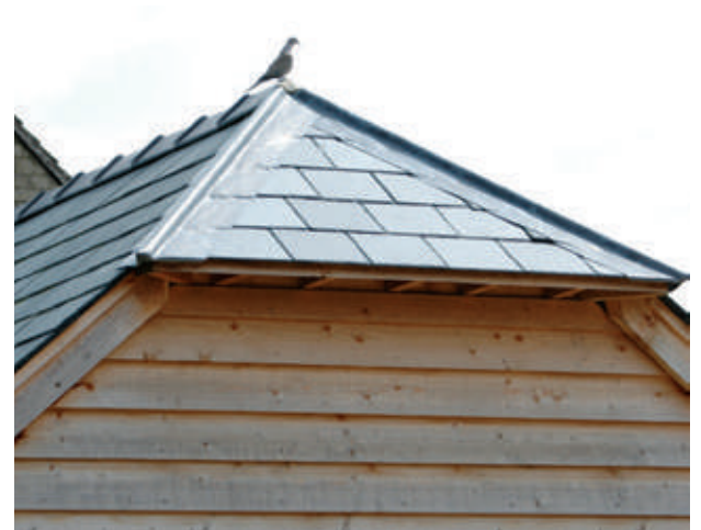
Slates with 'mopstick' lead hip detail
